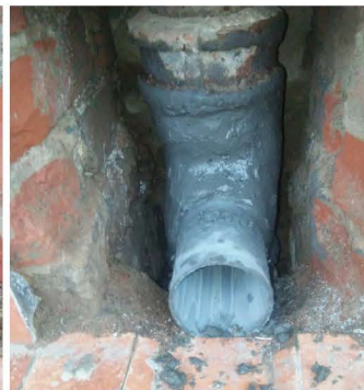
FOOTING DRAIN PART REPLACED
