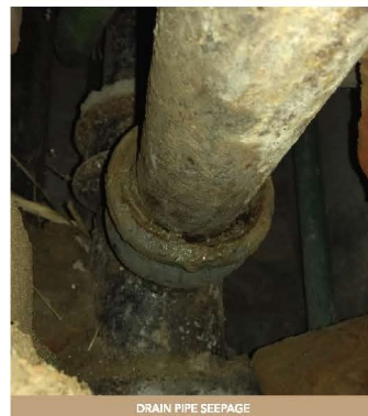
DRAIN PIPE SEEPAGE
