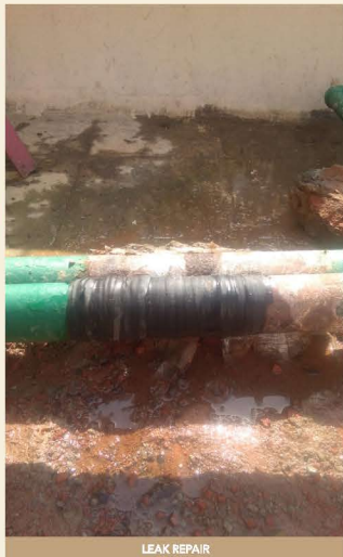
LEAK REPAIR
