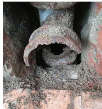
FOOTING DRAIN SEEPAGE
