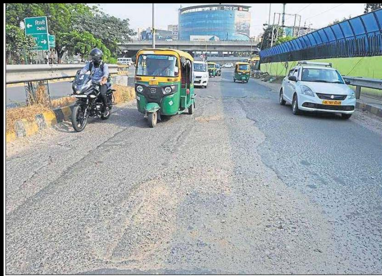
■ The Sector-17/18 dividing road was recarpeted in 2017, but the bituminous top layer came off within a year. The entire 2-km stretch is now covered in potholes.
